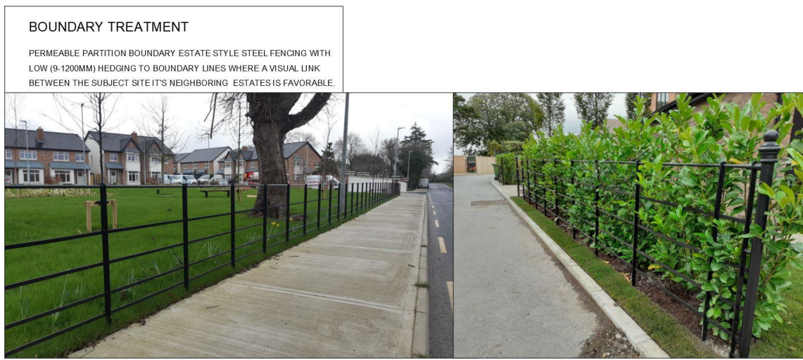
Fig. 17 – Permeable boundary detail Beech hedge & steel railings.
